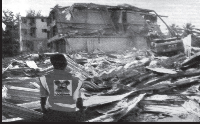
THE REMAINS OF THE COLLAPSED BUILDING AT MURI OKUNOLA STREET, VICTORIA ISLAND LAGOS.
