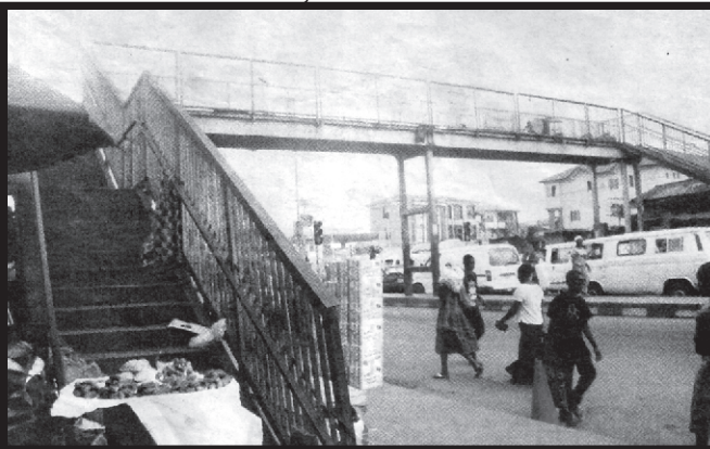
AN ABANDONED PEDESTRIAN BRIDGE TAKEN OVER BY ROADSIDE SELLERS AT OJUWOYE MARKET, MUSHINE, LAGOS
