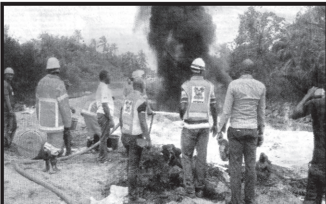
A scene of the Isegun Pipeline Explosion
