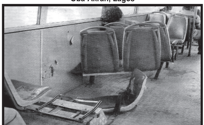
A failed section inside the Bus Rapid Transport in Lagos
