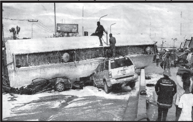
An accident scene of Daleko Bridge, Iyana-Isolo, Lagos State
