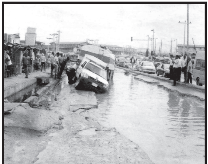
A BAD PORTION ON EJIGBO IKOTUN ROAD IN LAGOS
