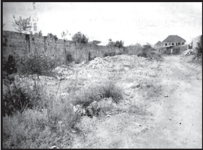
SCENE OF A DEMOLITION AT OKOTA, LAGOS
