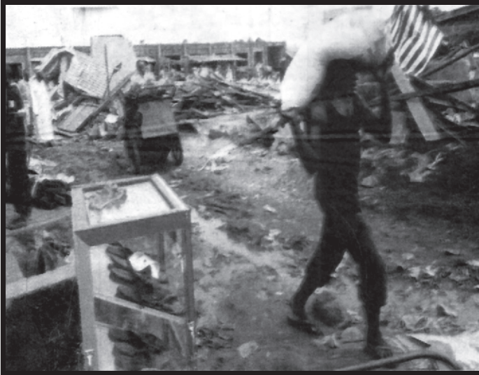
LAGOS ABATTOIR MARKET AFTER THE DEMOLITION
