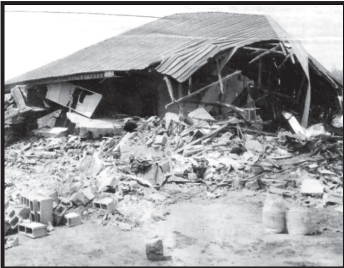
A DEMOLISHED BUILDING AT ATINPAROMOE AREA OF BADADRYIN LAGOS
