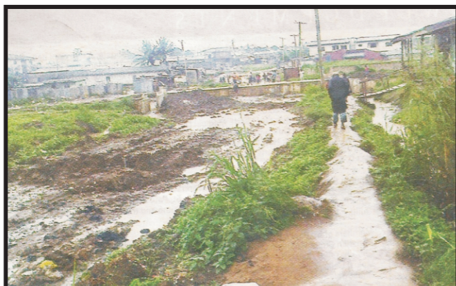
Abandoned Old Ota Road in Agbado Oke-Odo LCDA Lagos
