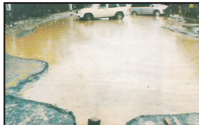
Flooded Baale Street at Orile-Iganmu after a downpour in Lagos
