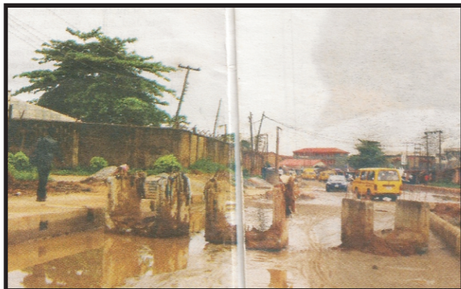
A section of Ipaja-Ayobo Road
